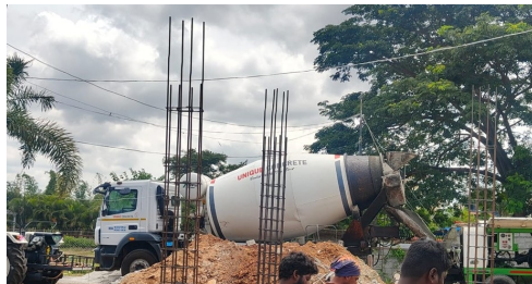
FOUNDATION & STRUCTURAL WORKS
